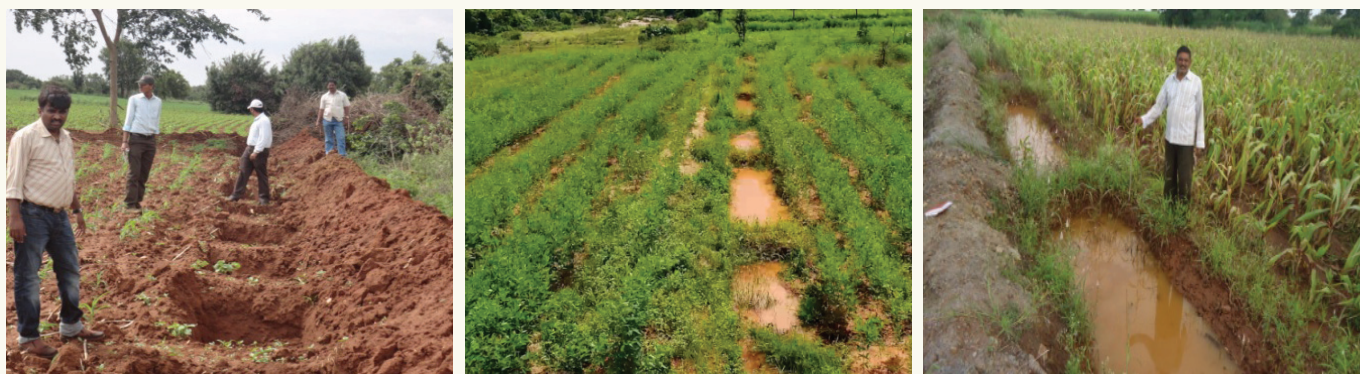
Trench cum bunds for soil moisture conservation and to increase the crop productivity during drought situations
